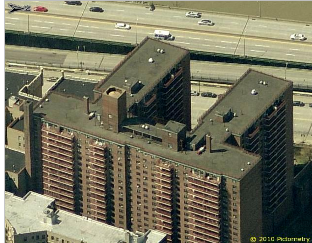
West Side View
