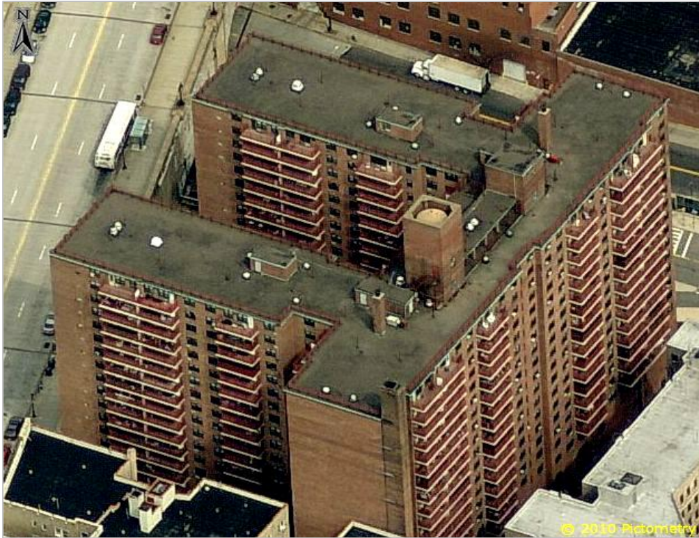
North Side View
